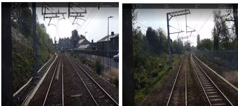
Figure 7-3: Vegetation clearance to support the Cardiff Queen Street Operation.
