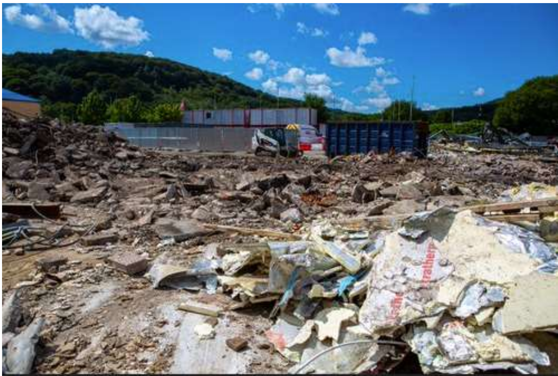
Figure 13-3: Taff's Well land developed – during demolition of site
