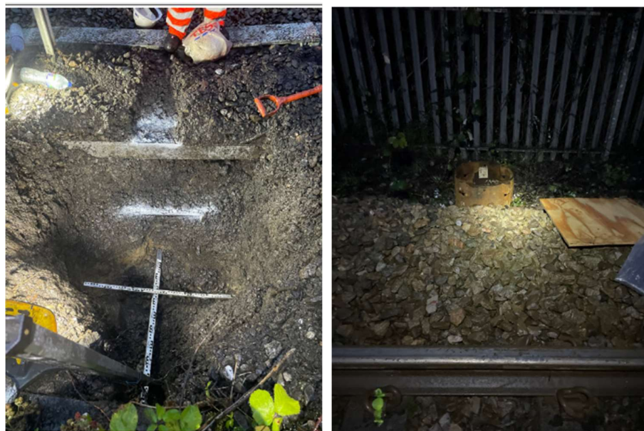
Figure 9-3: Overhead line equipment foundation installation on the Treherbert Line
