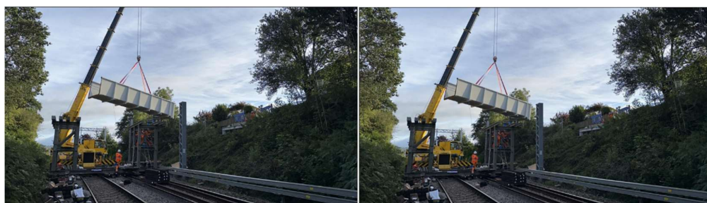
Figure 8-2: New footbridge at Lanks Hill, improving access to Danescourt Station
