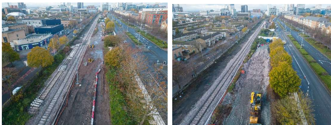
Figure 6-2: Cardiff Bay Stage 1 – track works adjacent to Lloyd George Avenue
