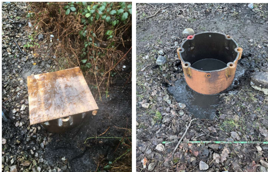
Figure 12-3: Overhead line equipment foundation installation on the Rhymney Line
