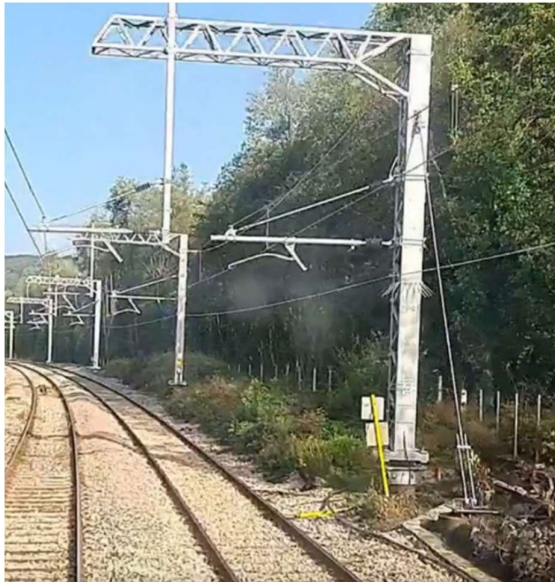
Figure 10-2: Overhead line equipment foundation installation at Aberdare
