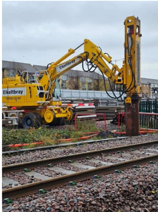
Figure 6-3: Cardiff Bay Stage 1 – preparatory works for electrification
