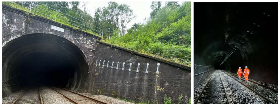
Figure 12-2: Caerphilly Tunnel works line speed improvements
