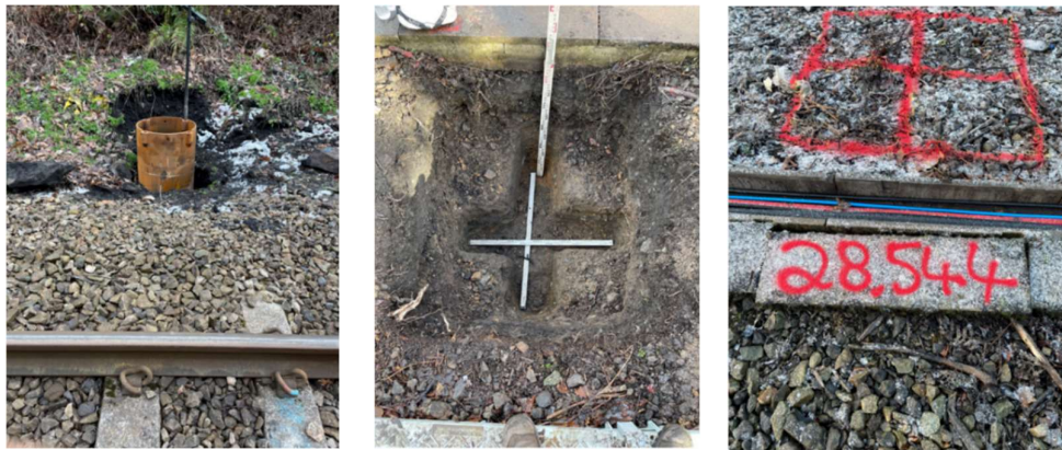
Figure 11-2: Overhead Line Equipment (OLE) foundations on the Merthyr Tydfil Line
