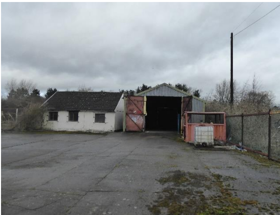
Figure M.7: Building B2 (Derelict 2)
