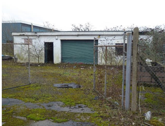
Figure M.6: Building B6 (Derelict 1)
