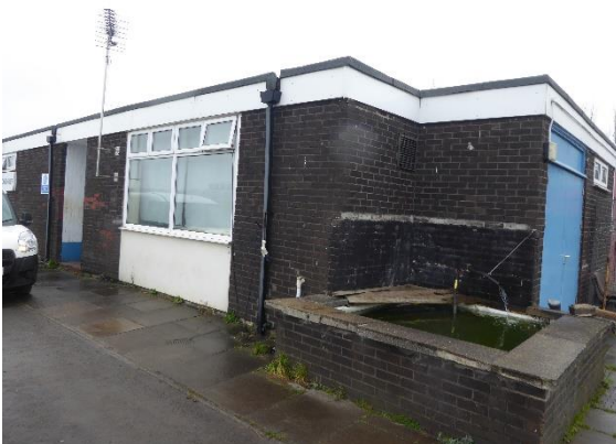
Figure M.3: Building B3 (DB Cargo)
