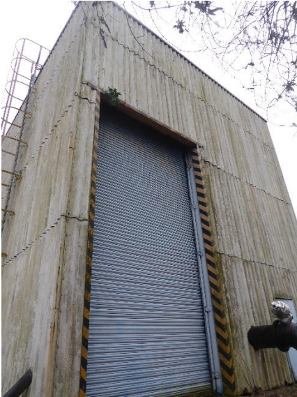
Figure M.1: Building B1 (Pumphouse)
