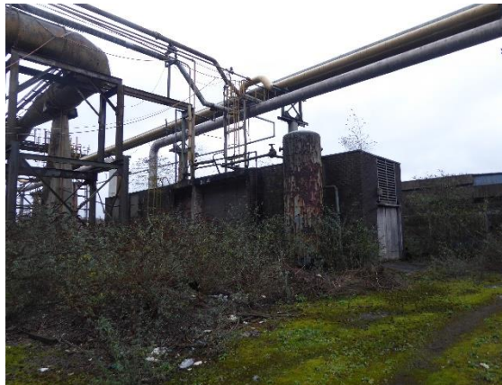
Figure M.8: Building B8 (LHS Building)
