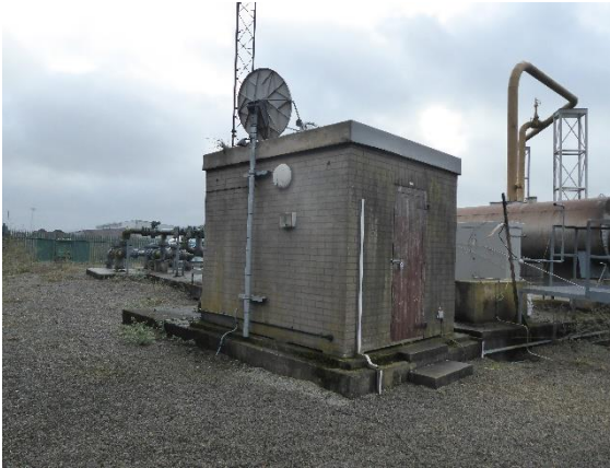
Figure M.5: Building B5 (Gas Station Associated)
