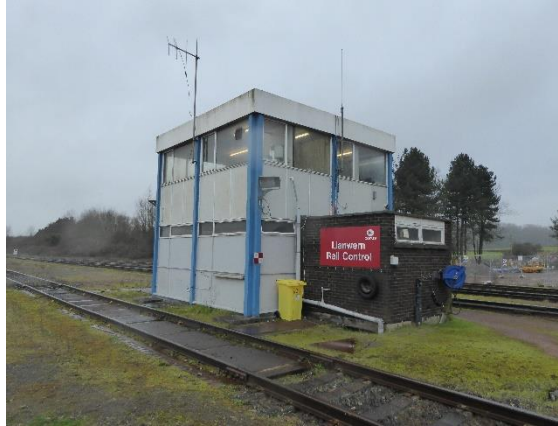
Figure M.2: Building B2 (Rail Control)
