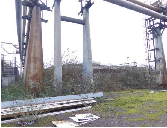
Figure M.9: Building B9
