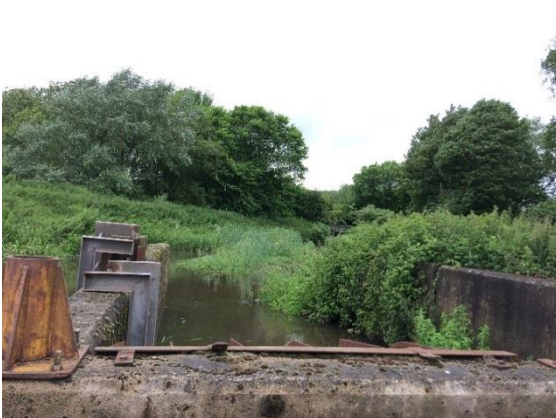
Photo 1: Monks' Ditch and Sluice gates
