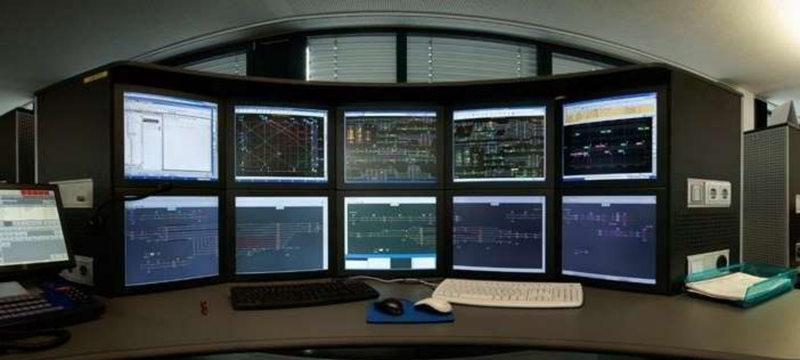
Rolling out Digital Rail - Traffic Management for the Central Metro and more of Wales (Newport to Shrewsbury)
